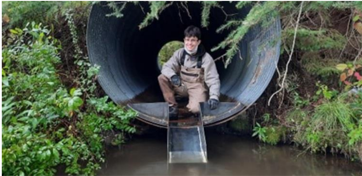
Figure 35: Outflow chute installed on Culvert C-017
