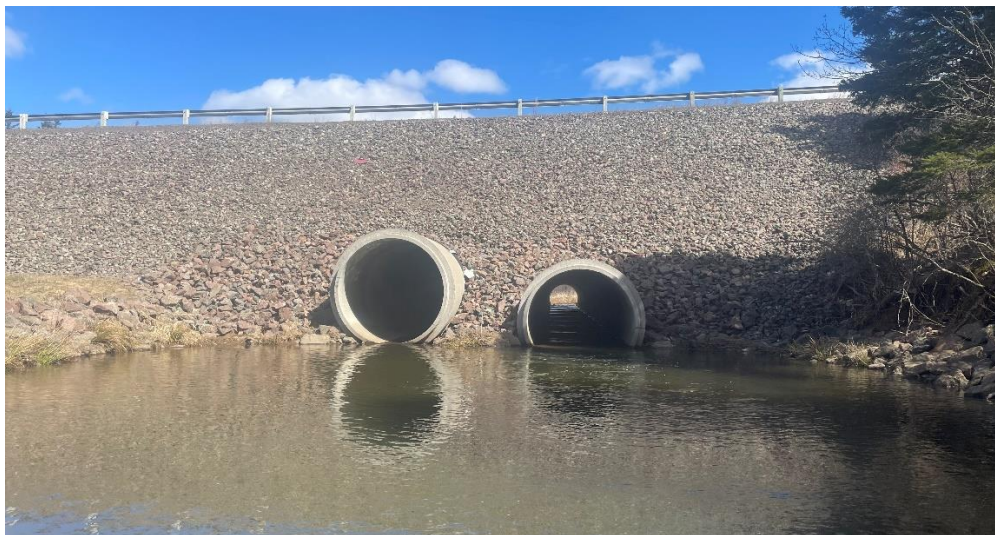
Figure 17: Outflow at new culvert on Route 126 in 2024
