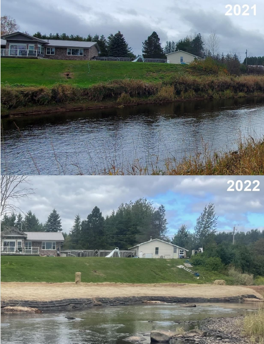
Figure 28: 2022 site before (2021) and after bank reconstruction (2022)
