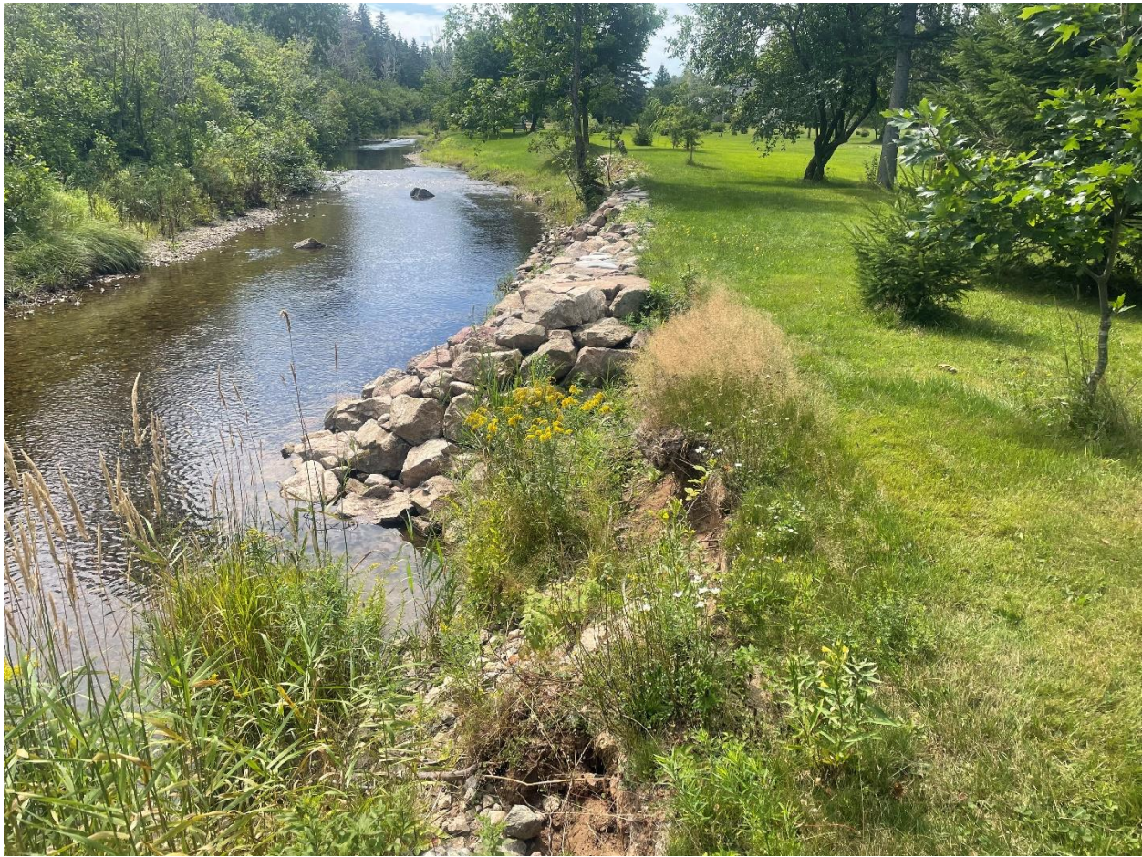
Figure 36: Riprap hardened bank upstream of the 2023 project
