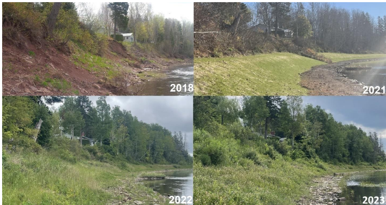
Figure 28: Bank Restoration at Highland Park from upstream looking downstream 2018 to 2023.
