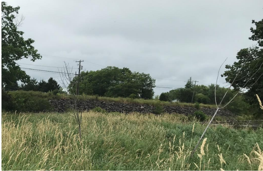
Figure 24: Riprap armoured bank below Route 106
