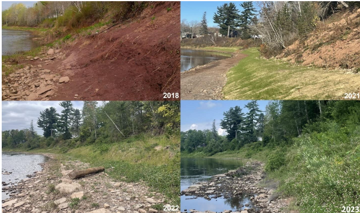
Figure 29: Bank Restoration at Highland Park from downstream looking upstream 2018 to 2023.
