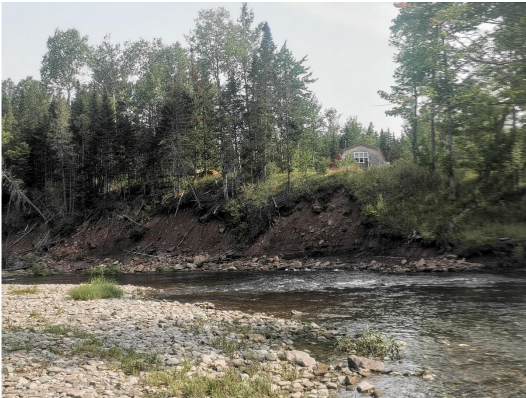
Figure 18: Aggradation (gravel bar) in Reach 60 promoting widening (bank failure) in Reach 61
