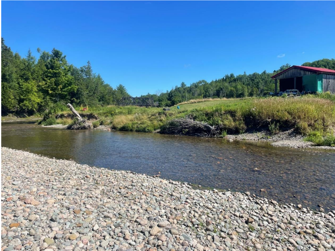
Figure 40: Failing section of riverbank near Elgin planned for 2025 Bank Restoration Project
