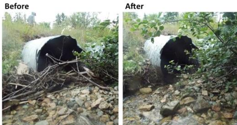
Figure 31: Before and after photos of C-022, located where Church Hill Road crosses Sheffer Brook
