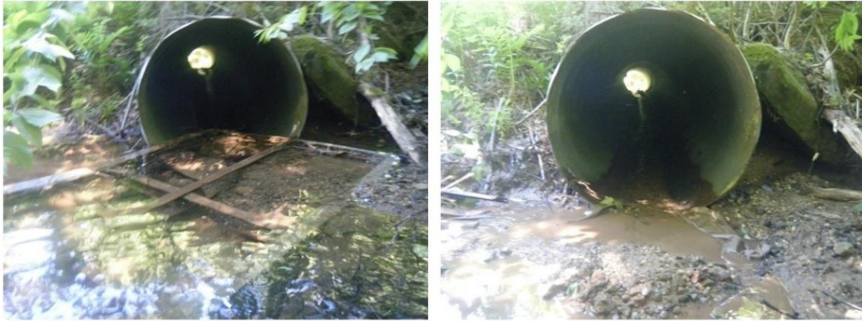
Figure 4.5 Culvert C-172 before and after PWA removed debris including a mattress in 2017
