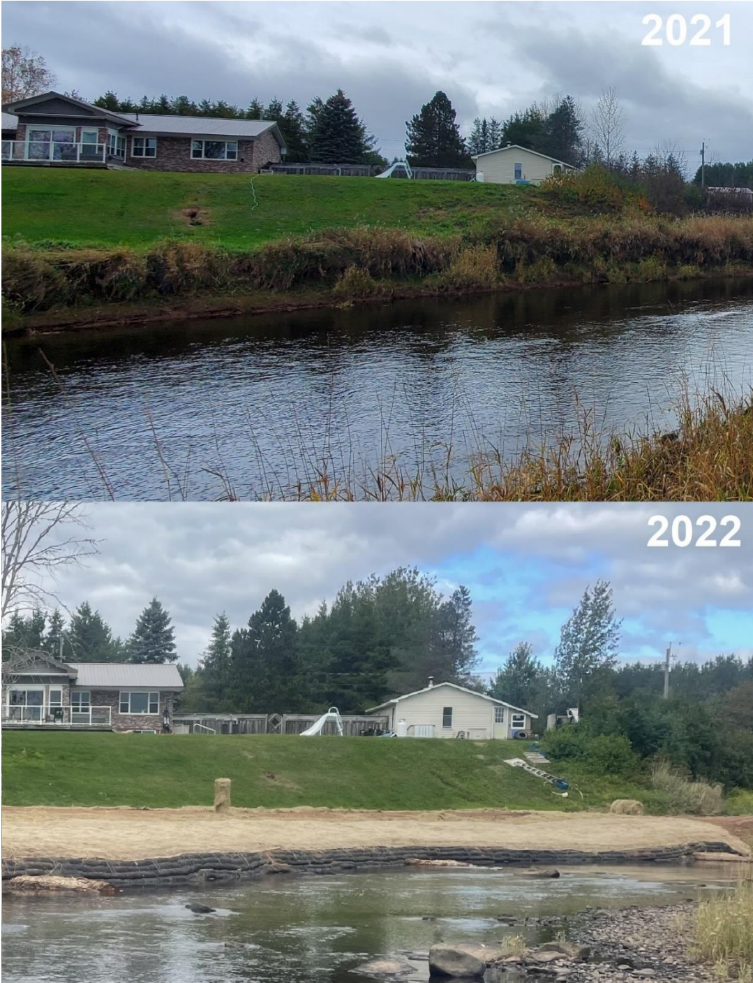
Figure 28: 2022 site before (2021) and after bank reconstruction (2022)
