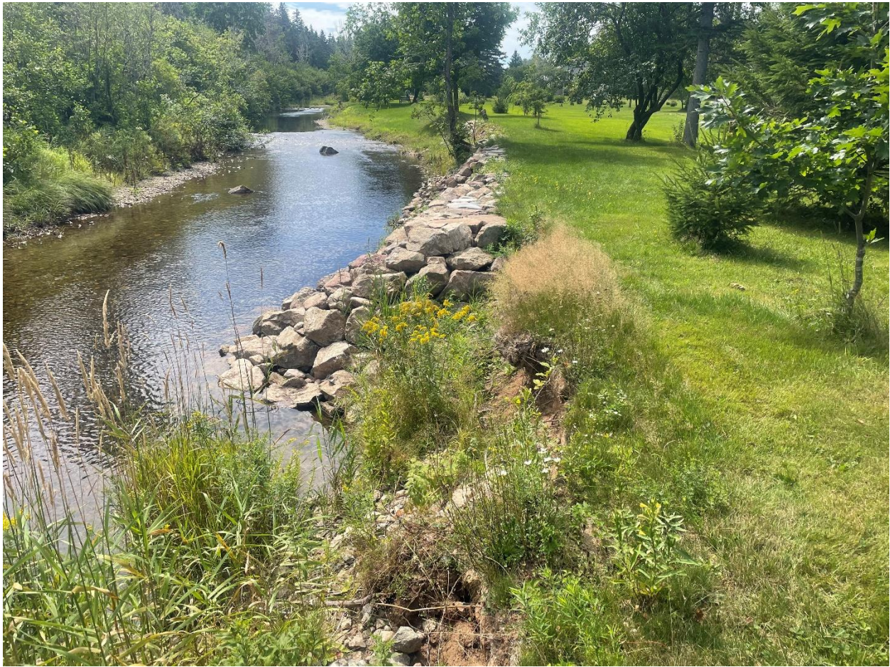
Figure 36: Riprap hardened bank upstream of the 2023 project
